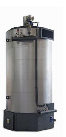
We design and manufacture recuperators for heat recovery for different types of industrial and marine applications. Our recuperators use exhaust fumes from motors, electric generators, ovens, incinerators and other industrial processes and transfer heat to a secondary fluid, which can be steam, water, diathermic oil or even air.
