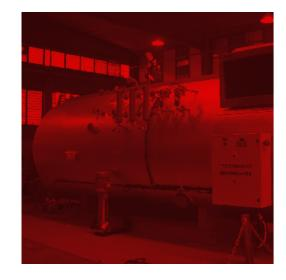
The model GPT is a 3-passes boiler with wet back wet. It can produce from 3,000 to 25,000 kg of steam per hour with a pressure up to 21 barg. It's used both for liquid and gaseous fuels and it allows a two-position regulation or in a modulating version both on fuel and on feed water.
